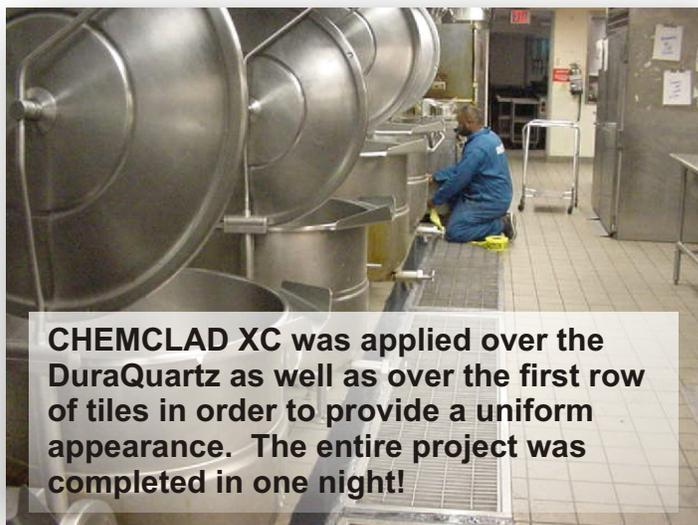
CHEMCLAD XC was applied over the DuraQuartz as well as over the first row of tiles in order to provide a uniform appearance. The entire project was completed in one night!
