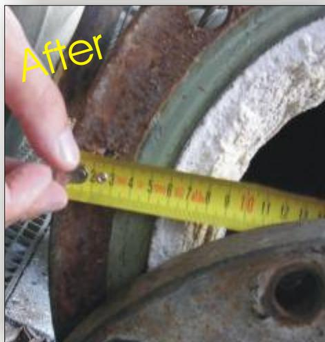
The maintenance engineers at this large power station - one of the biggest - in Poland had been experiencing a very severe mineral (lime) scale problem in their cooling water lines which carry water from a nearby lake. This scaling was so severe that it often rendered the pipes "useless" necessitating extensive cleaning or replacement.
