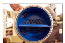
These heat exchangers at a Silicon Valley data center circulate reclaimed water, which contributes to accelerated erosion and corrosion.
